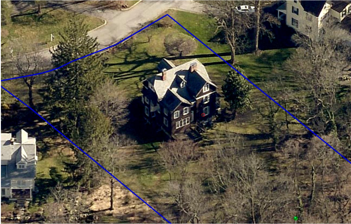
Exhibit 6: Aerial view east elevation 2020 Pictometry
